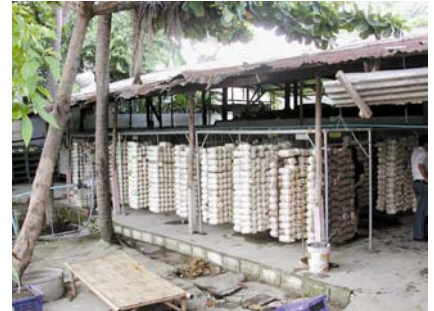
Figure 6. Steel frame structure with a roof
