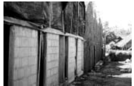
Figure 9. Steam pipes on the brick wall
