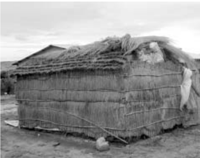
Figure 23. Growing house at Mbangweni
