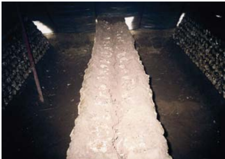
Figure 4. The walls shown from above
