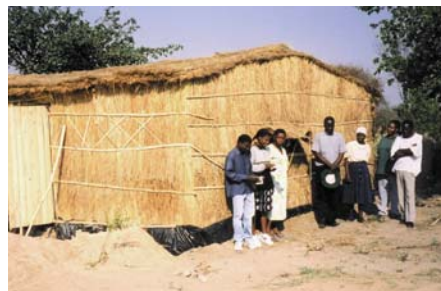
Figure 12. Rodent/snake barrier in the bottom part (Photo courtesy of Audrey R.S Mabveni)
