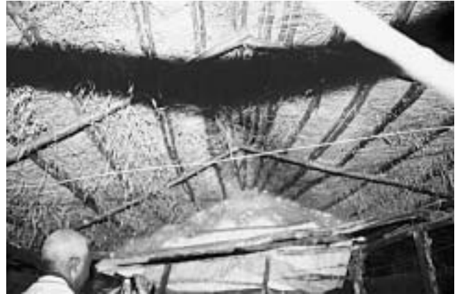
Figure 26. Inside growing room made by logs and grass-the roof
