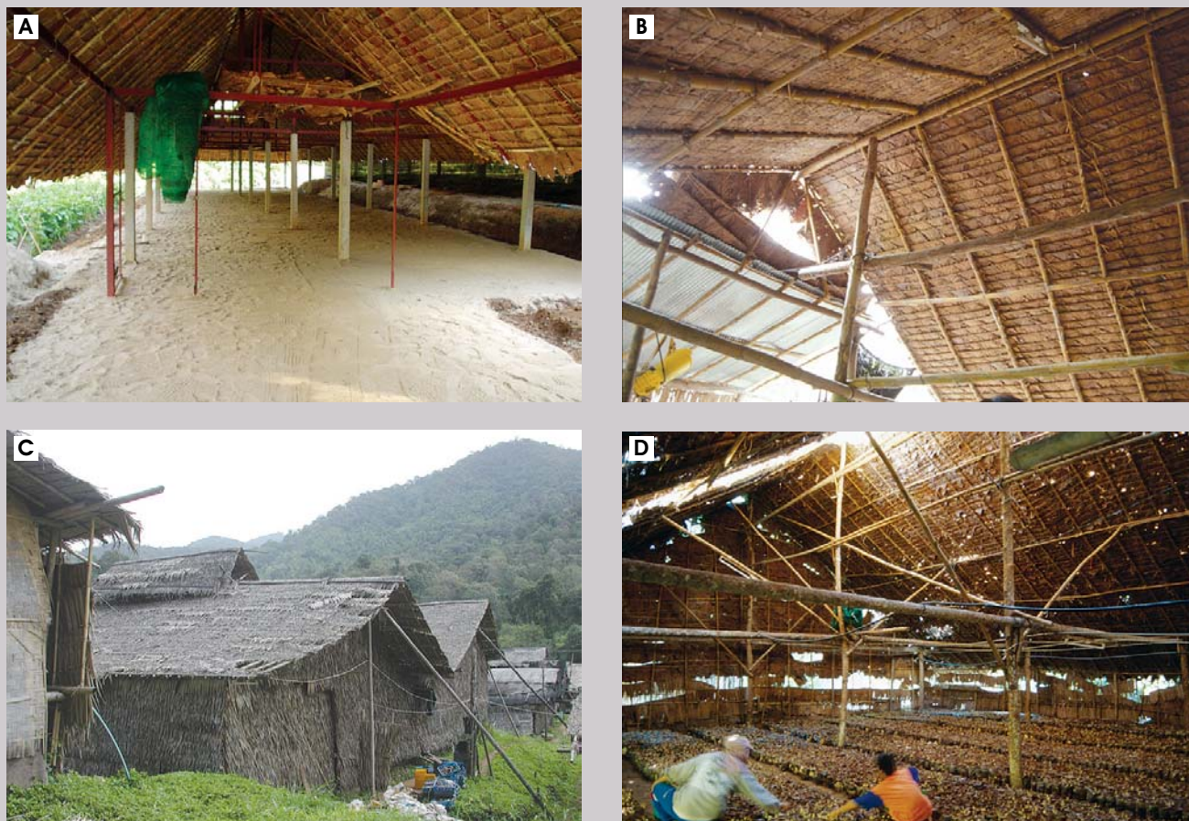
Figure 5. Recommendations for better growing houses A: Floor covered with sand B: High roof to prevent heat accumulation C: Ventilation opening on the roof D: Wall made of only local leaves
