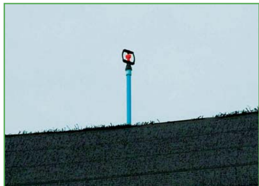
Figure 12. Sprinkler on the roof (Photo courtesy of Tawat Tapingkae)
