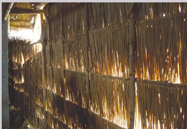
Figure 15. Light leaking into growing house
