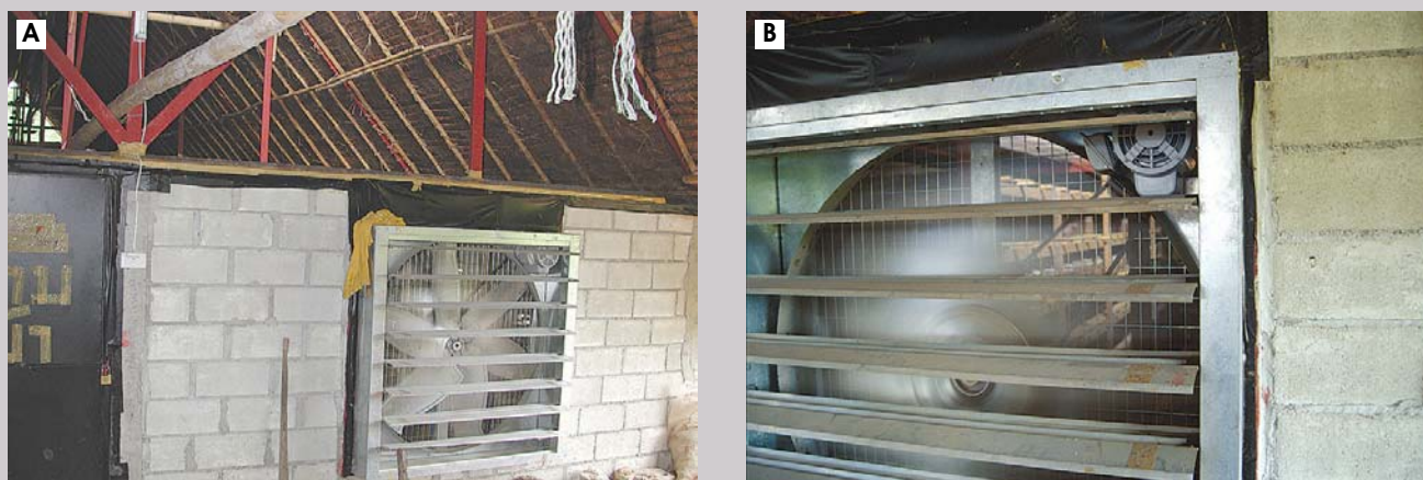
Figure 8. Incubation room with controlled system A: Separated incubation room equipped with "fan and pad cooling system" B: Shiitake bags under spawn run on shelves (seen through a big fan on the wall)
